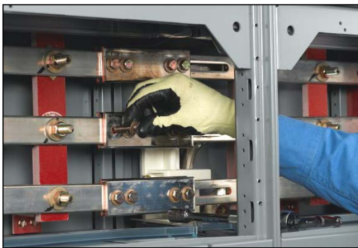
Figure 45: Inserting the Splice Bolts
