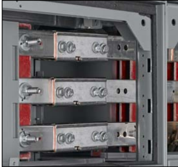
Figure 51: Removing the Bolts from the Splice Assembly
