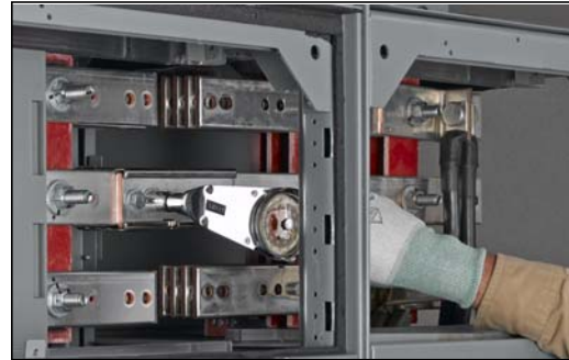
Figure 55: Torque All Bolts
