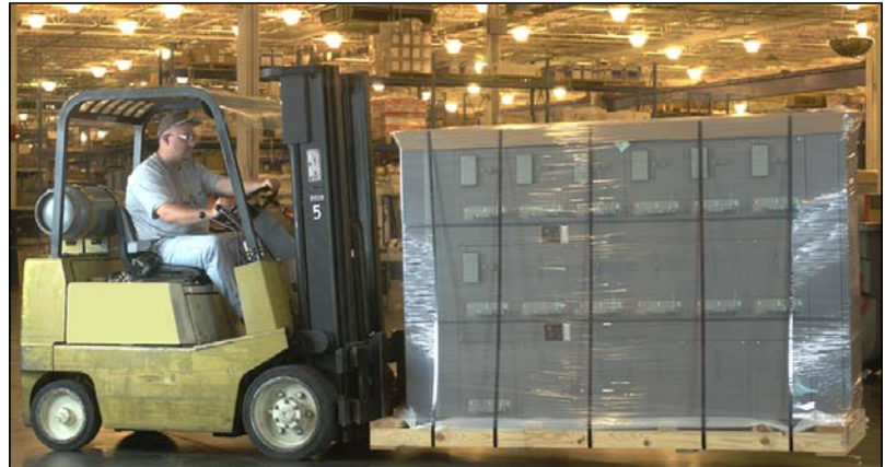
Figure 4: Moving the MCC with a Fork Truck
