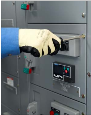
Figure 85: Loosening Captive Fasteners
