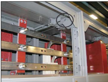
11F: Top Front Side Channel Connection
