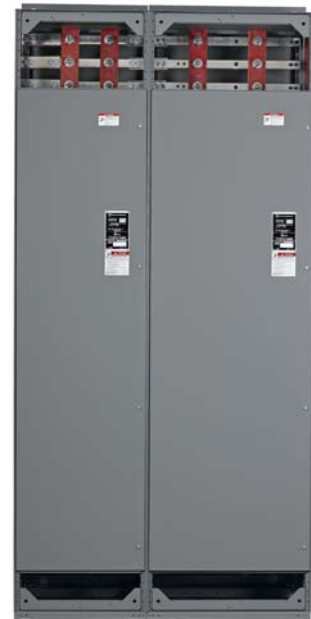
Figure 8C: Two-piece Bus Barriers Removed (splice connection made)
