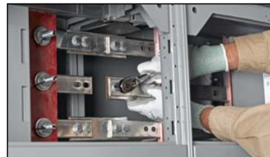
Figure 31: Removing Bolts from Single-Splice Bar
