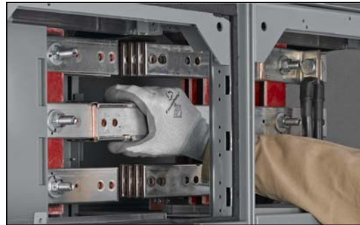
Figure 52: Aligning the Splice and Bus Holes
