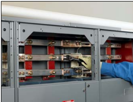
Figure 43: 85,000 A Bracing Option
