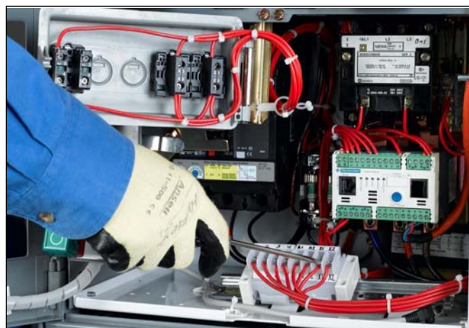
Figure 63: Pull-apart Type Terminal Blocks
