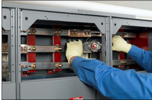
Figure 40: Torquing the Bolts
