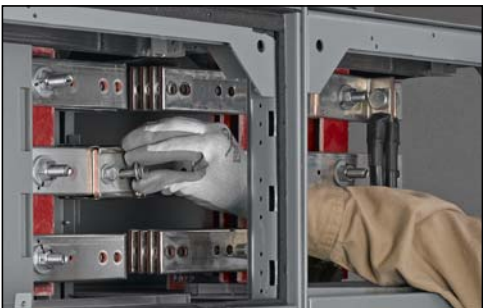
Figure 53: Inserting the Splice Bolts
