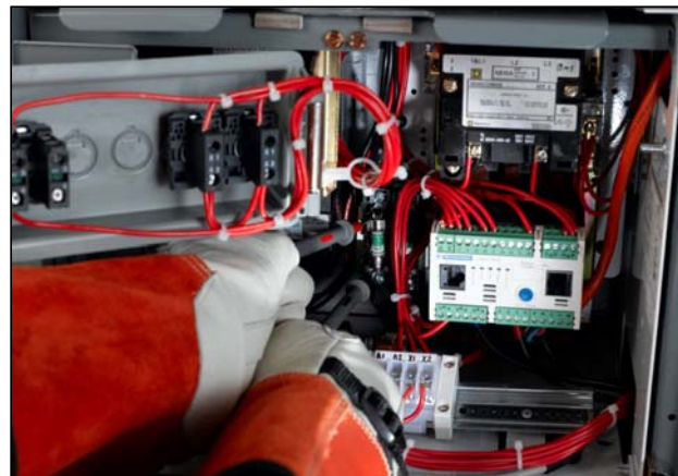
Figure 90: Inspecting Fuses
