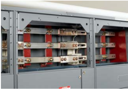
Figure 42: Loosen Bolts
