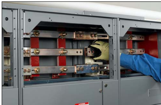
Figure 37: Aligning the Splice and Bus Holes
