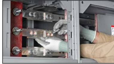
Figure 32: Moving and Aligning the Splice Bar to the Bus Holes
