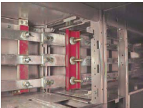
Figure 43: 85,000 A Bracing Option
