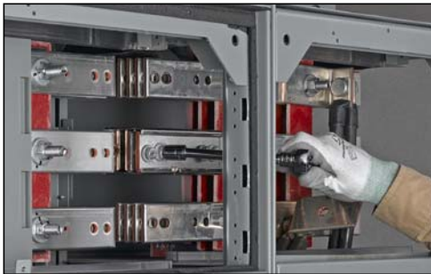
Figure 51: Removing the Bolts from the Splice Assembly
