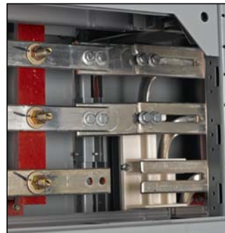
Figure 30: Incorrect Application of Single-Bar Splice on Fork-Type Bus
