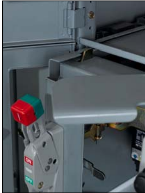
Figure 79: Operating the Mechanism-to-Structure Interlock
