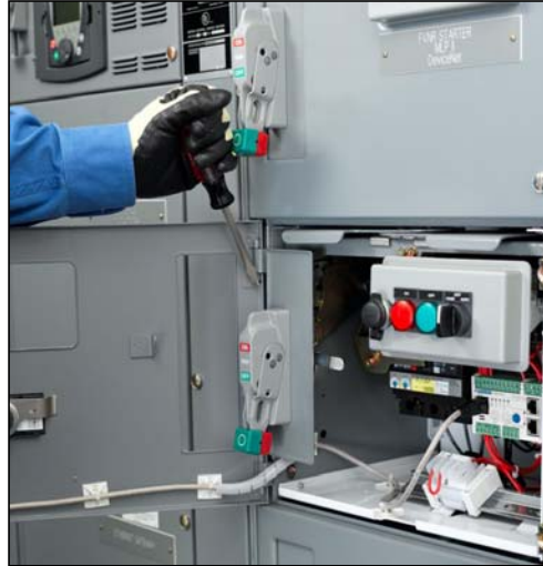
Figure 83: Driving Out Hinge Pin
