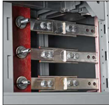
Figure 30: Incorrect Application of Single-Bar Splice on Fork-Type Bus
