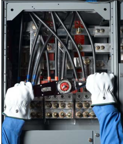
Figure 66: Main Lug Compartment Torque Connection
