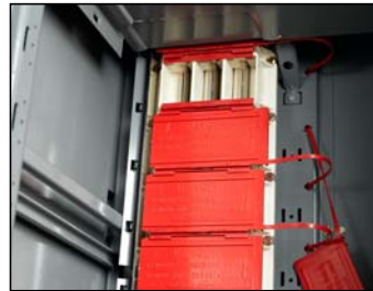
Figure 118: Removing the Manual Bus Shutter
