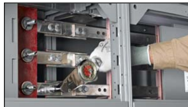
Figure 35: Torquing the Bolts
