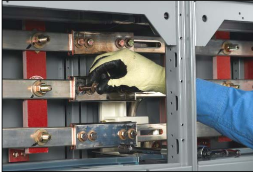
Figure 38: Inserting the Splice Bolts
