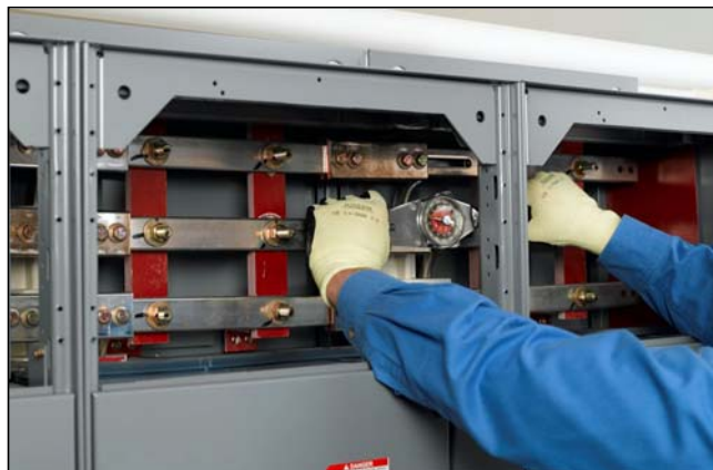
Figure 47: Torque All Bolts
