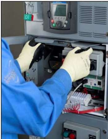
Figure 119: Engaging the Cam Mechanism
