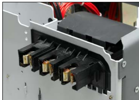
Figure 88: Stab Assembly
