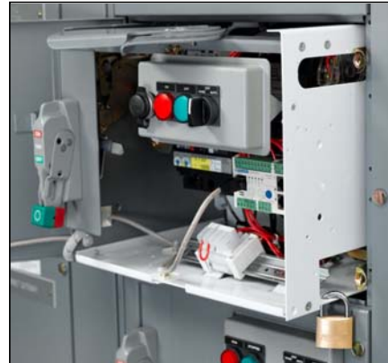
Figure 80: Locked Out Device
