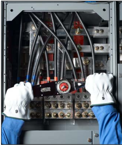
Figure 70: Main Lug Compartment Torque Connection
