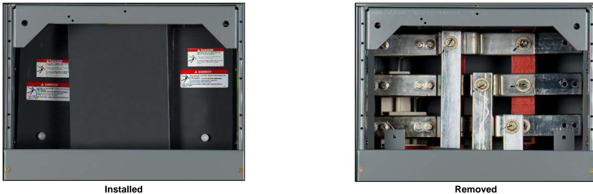
Figure 134: Barrier Installed and Removed
