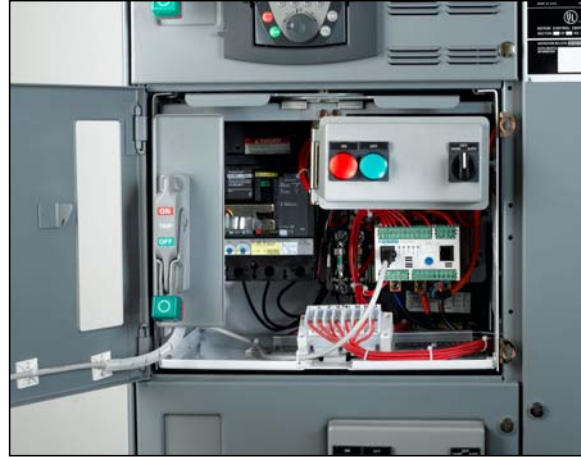
Figure 113: NEMA Rated Control Unit (TeSys T Modbus)
