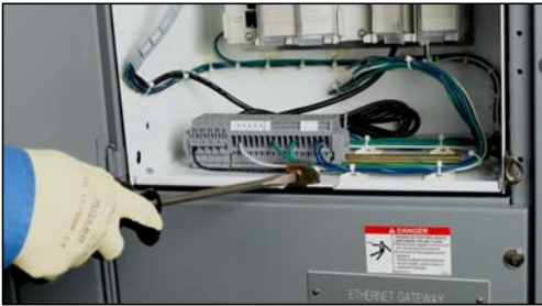
Figure 75: Releasing the Lock-in Device (when supplied)
