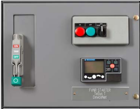
Figure 72: Operator Mechanism in the OFF Position
