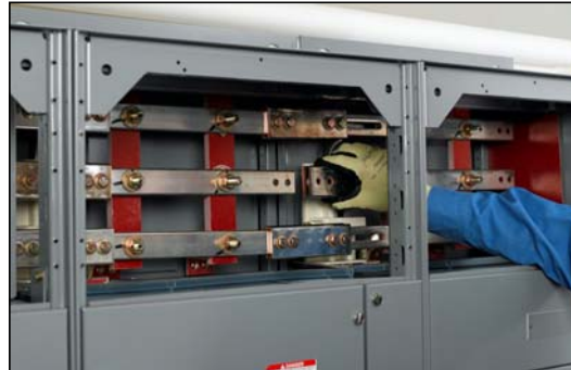
Figure 44: Slide the Splice Assembly to the Left
