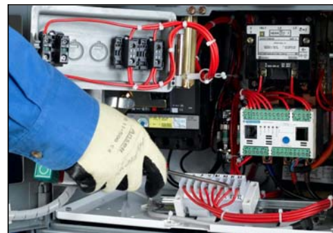
Figure 123: Connecting Control Leads to the Terminal Blocks
