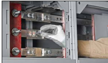
Figure 34: Placing a Conical Washer Under the Bolt Head
