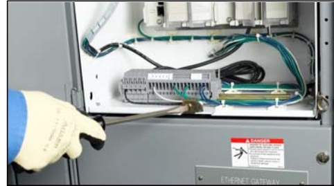
Figure 121: Tightening the Control Unit Lock-in Panel (when supplied)
