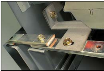
Figure 49: Ground Bar Bolt Replaced
