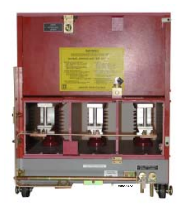
Figure 19: Temporary Ground Cables Removed
