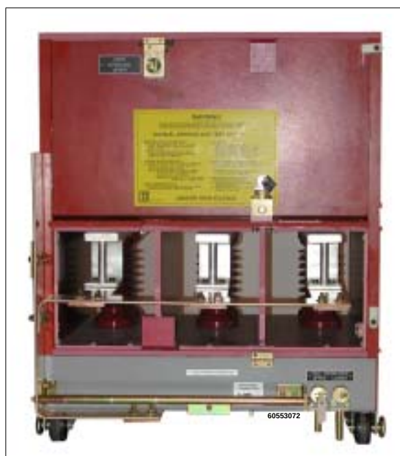
Figure 35: Temporary Ground Cables Removed
