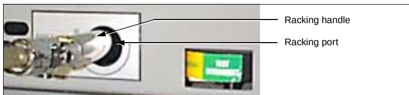
Figure 44: Racking Handle Engaged onto Racking Shaft with Circuit Breaker in the TEST/DISCONNECT Position
