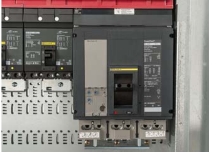
Powerpact P-Frame 1200 A Main (the maximum size circuit breaker for the I-Line Combo panelboard)
