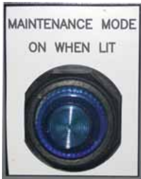
Figure 8: Local Maintenance Mode Indicator Light
