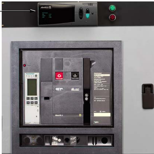
Figure 21: Powerlogic Circuit Monitor Display
