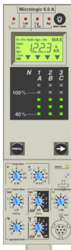
Micrologic Type A Trip Unit
