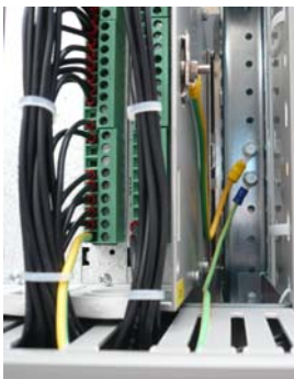
Correct (short connection with 1.5 mm 2 to the common grounding point of the cabinet (Not illustrated: Incorrectly mounted with long lead in the cable harness together with conductors from the transformers etc.)
