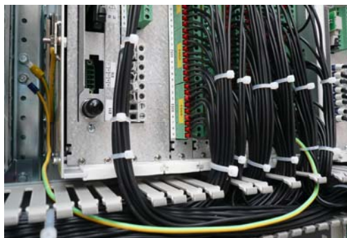
Correct (short connection with 1.5 mm 2 to the common grounding point of the cabinet (Not illustrated: Incorrectly mounted with long lead in the cable harness together with conductors from the transformers etc.)
