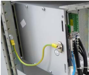
Correct (short wire 2.5 mm 2 )
