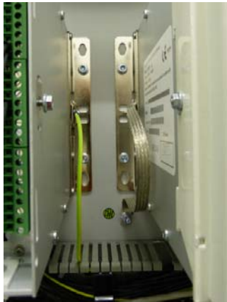
Correct: Wire or copper braid
