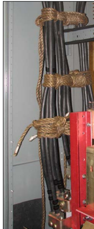
Figure 25 – Cable Restraint Example
