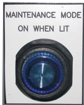
Figure 8 – Local Maintenance Mode Indicator Light
