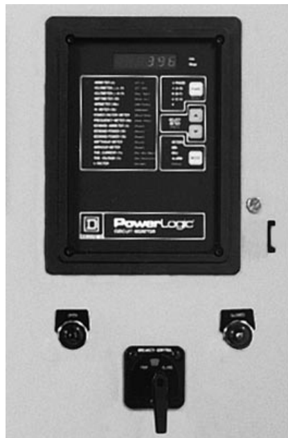
Figure 1. In addition to its primary power monitoring functions, the PowerLogic® Circuit Monitor can be used for ground fault detection.
