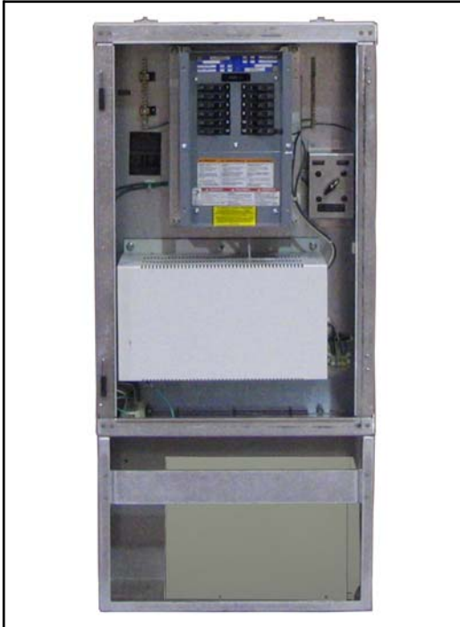
Figure 29: Power Manager with Optional Battery Back-up
