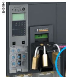
Toggle locked by removable padlocking device
