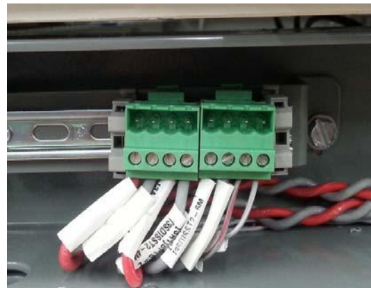
Figure 42: Modbus RS485 Stationary Connector in Left Side of Bottom Front Wireway
