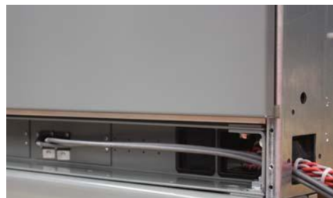
Figure 40: ULP Cables routed and connected to labeled ULP ports in adjacent section wireway
