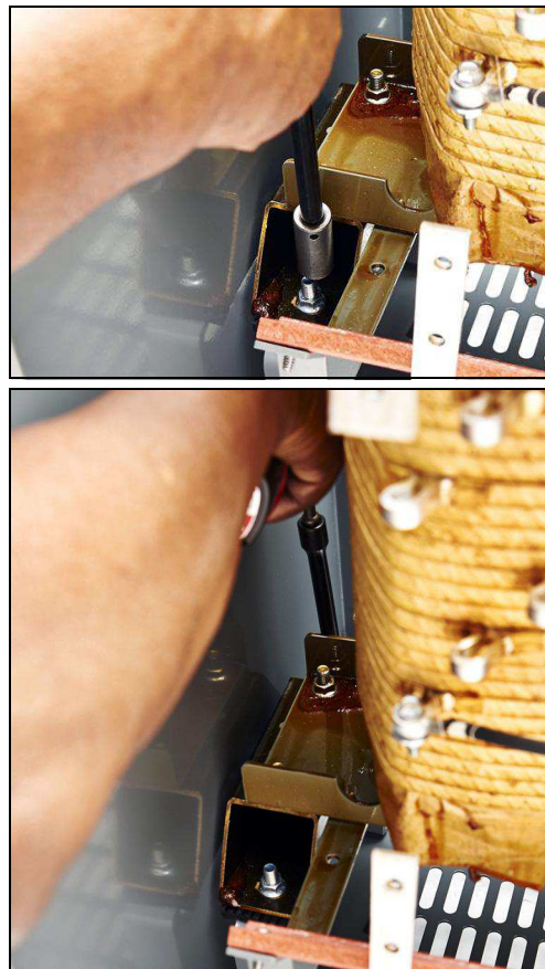
Figure 27: Enclosure Style K: Bolts Accessible from the Front of the Transformer
