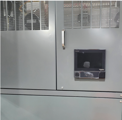
Figure 13 - QED-2 with ION9000 Meter with Optional 7 in. Color Touchscreen Display
