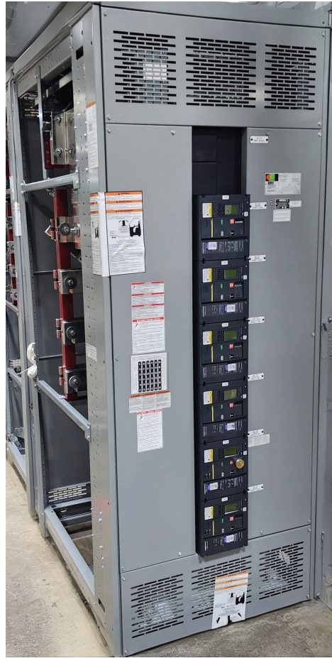
Figure 3 - QED-2 I-Line Section with Bus
