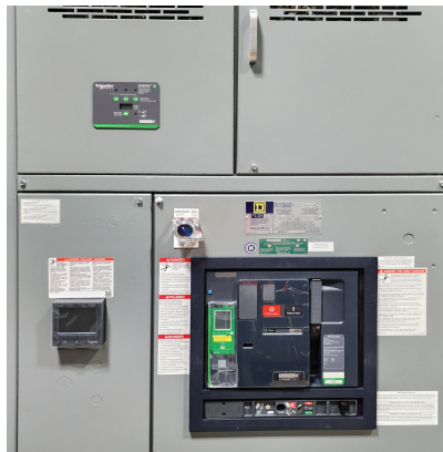
Figure 9 - 2000 A MasterPacT™ Main Circuit Breaker with PowerLogic Power Meter
