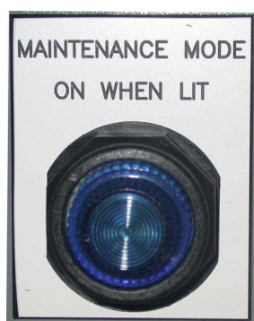
Figure 8 – Local Maintenance Mode Indicator Light
